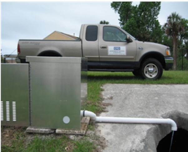
c. Housing for Sample Tubing and Flow Probes
